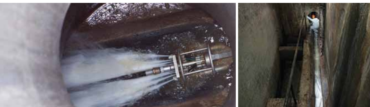
Far left: High-pressure water cleaning systems are used to clean sewers with the diameter of up to 1100 millimeters.
